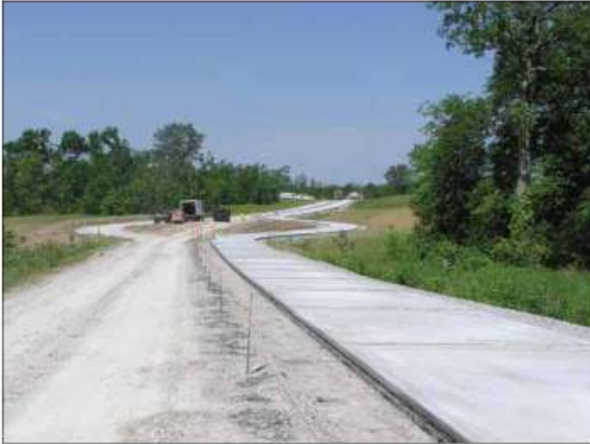
The concrete project required low-impact construction to stay within environmental guidelines.
