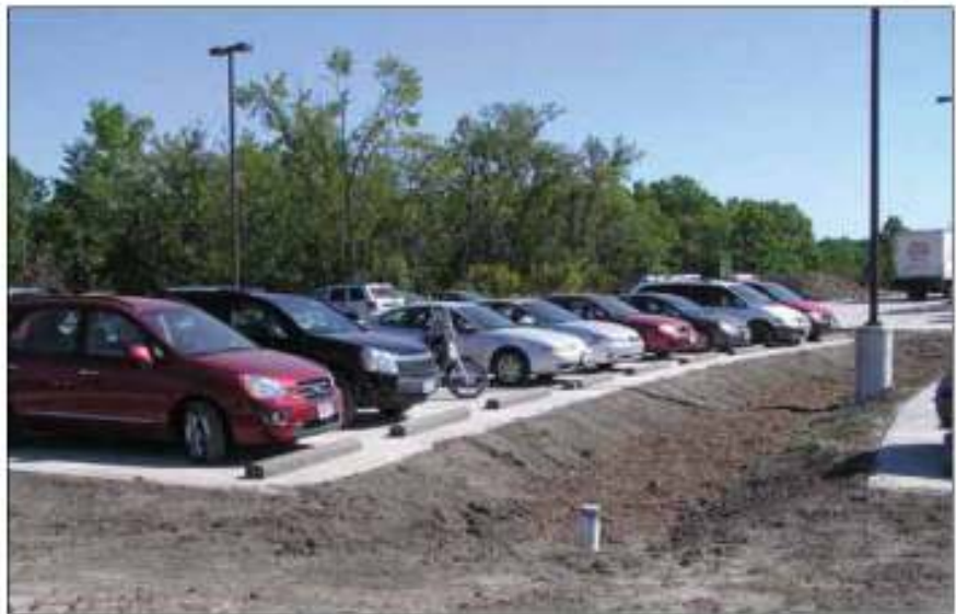
Bioswales, such as the one shown to the right of this finished concrete pavement, act to remove contaminants in the parking area before rainwater runoff can reach the lake, which is immediately behind the lodge. Excess rainwater then percolates into the ground in the bioswales.
